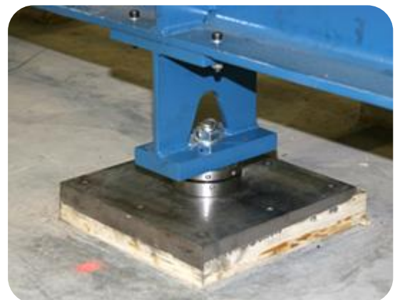
Chocking of the structure
