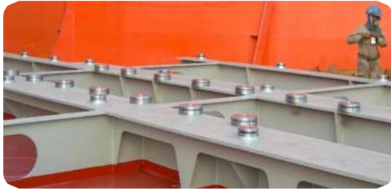
Preparation of compressor set chocking
