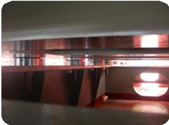
Compressor set chocked and mounted
